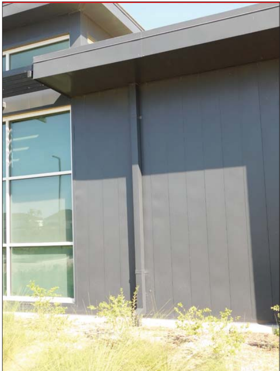
Roofing - Typical roof gutter and downspout
