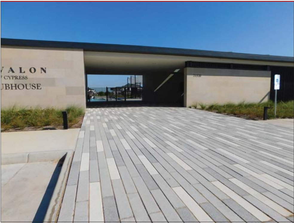
Painting & Repairs - Clubhouse entryway pavers
