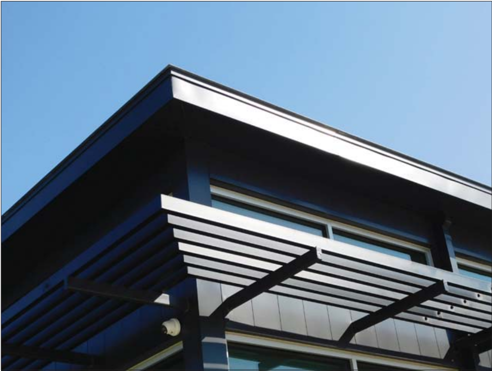
Roofing - Typical metal roofing
