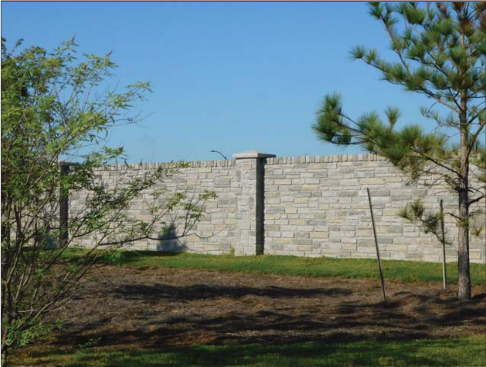
Fences & Walls - Typical perimeter masonry wall
