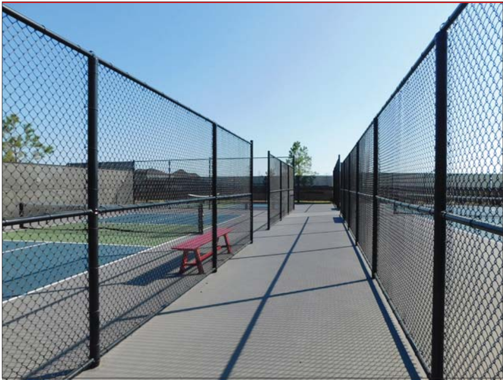
Fences & Walls - Chain-link fencing
