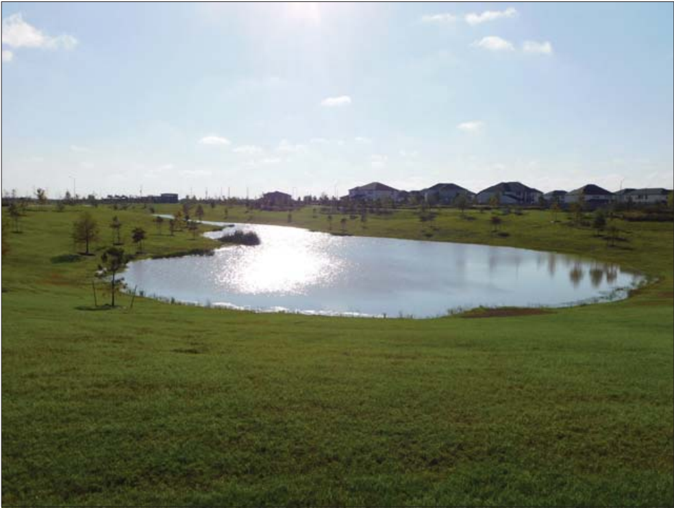
Drainage & Irrigation - Stormwater pond
